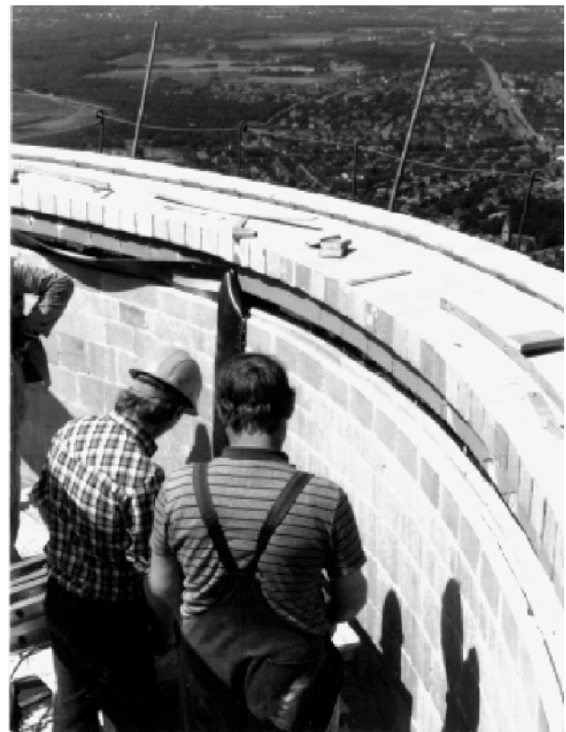
Technicians installing a lining joint sealing.
