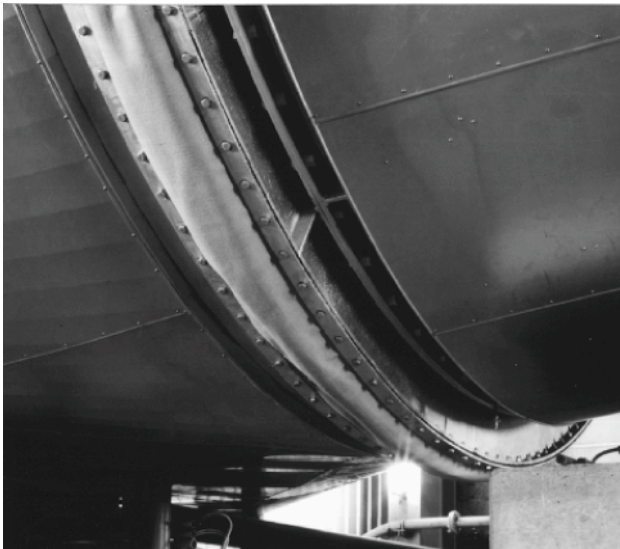
KLINGER Kempchen compensators in flue gas distributing main
